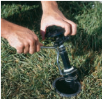
1. Remove internal assembly of existing sprinkler.
