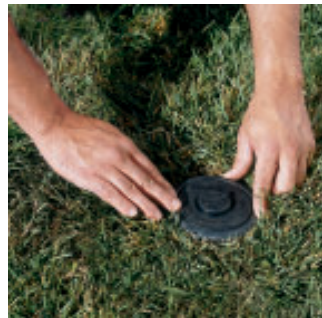
Install Cap portion of ATR, or to make it invisible, fill cup with sod.
