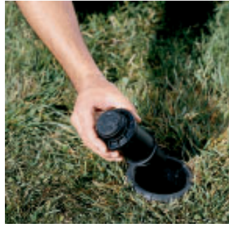
2. Thread entire ATR body/riser into canister.
